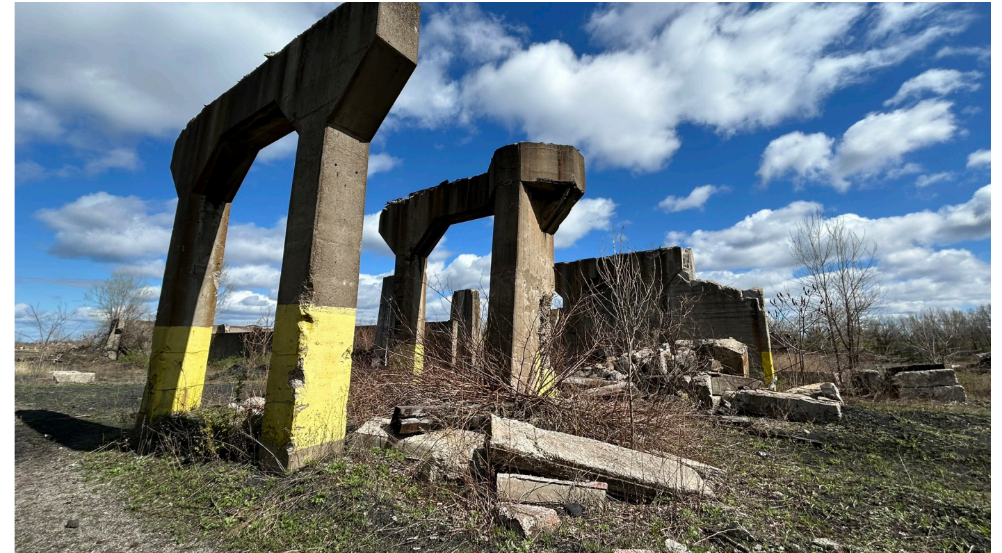
Figure 21: Remnants of the Coke Plant on the former Erie Coke Site
