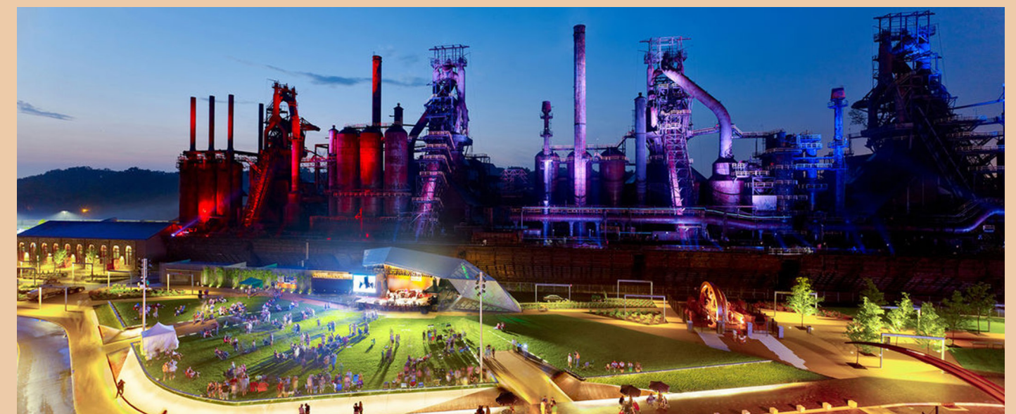
Figure 79: Bethlehem Steel Works, Source: WRT Planning + Design
