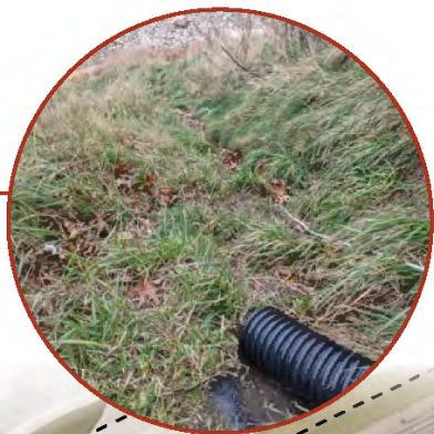
A rill is forming from the discharge of a drainage pipe at the top of the slope. Moving the pipe down the slope and discharging at the toe is preferred.
