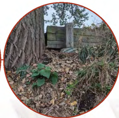
Steep bluff slope crests right at the edge of the walkway. Erosion is undermining the walk and causing it to tip down the slope. Wood retaining wall measures have been put in place at locations.
