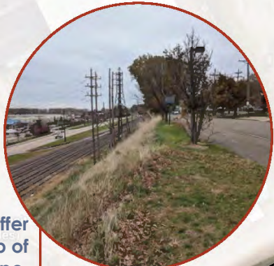
Steep bluff slope crests right at the edge of the walkway. Erosion is undermining the walk and causing it to tip down the slope. Wood retaining wall measures have been put in place at locations.
