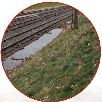
A swale holds water and debris along the majority of the bluff at the toe.
