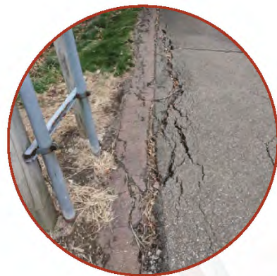
Steep bluff slope crests right at the edge of the walkway. Erosion is undermining the walk and causing it to tip down the slope. Wood retaining wall measures have been put in place at locations.
